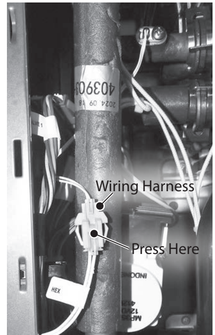
Figure 76 - Wiring harness location
