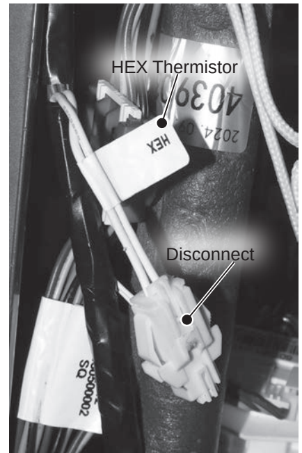
Figure 43 - Disconnecting HEX thermistor
